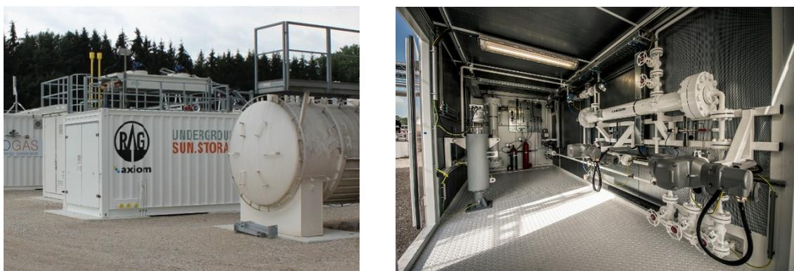
**Figure 5: hydrogen separation unit using based on a one-stage membrane gas permeation system constructed within the Underground Sun Storage project**
